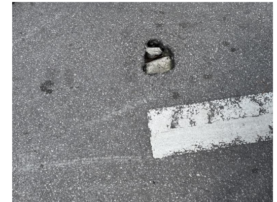
Figure 2: Some parts of PPR Beringin have also shown signs of other physical hazards, such as land subsidence and minor sinkholes, which may be linked to prolonged water seepage and poor soil stability beneath paved surfaces.
