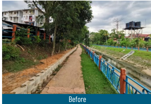
Figure 3.72: Before and After Installing Vertical Green System (VGS) along Sg Bonus in Wangsa Maju Seksyen 1
