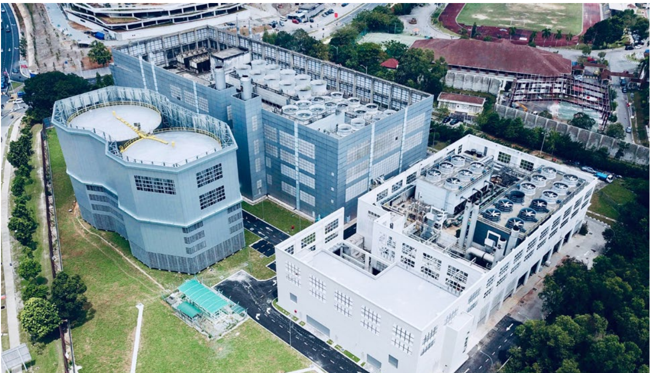
Gas District Cooling (GDC) Plant 1, Putrajaya
