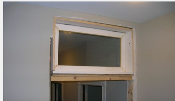
Windows above interior doorways
