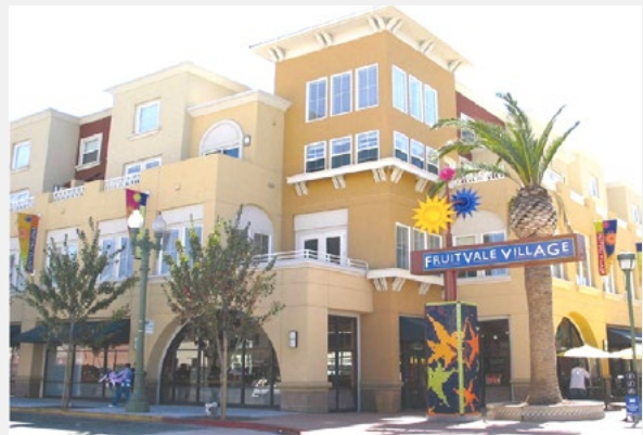
Two building, mixed use, transit oriented development that gives train passengers to the Fruitvale neighborhood.
